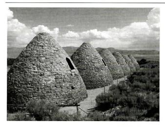
Figure 2. The Ward charcoal ovens. Each oven is approximately seven meters tall and nine and a half meters in diameter.
