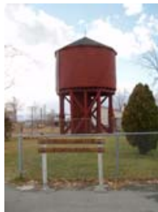
Rehabilitated Gerlach Water Tower
