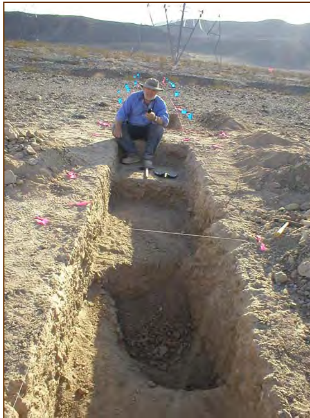
A plaintive Claude pondering the excavation units on the Kern River Pipeline Expansion Project 2001.
