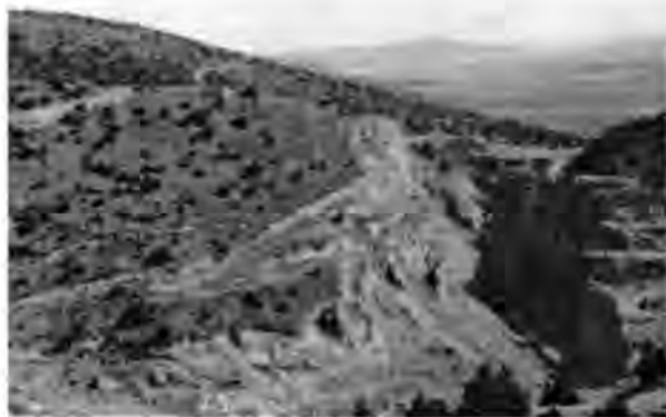
Figure 3. Overview of a portion of the Lally Pit. Note the scars on the lower right hand side of the photograph. These are fault scarps created during the slide.
