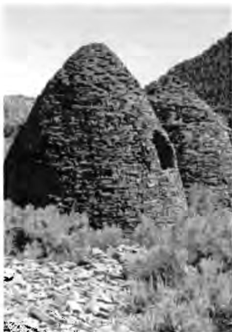
Figure 2. Beehive-shaped charcoal oven.
